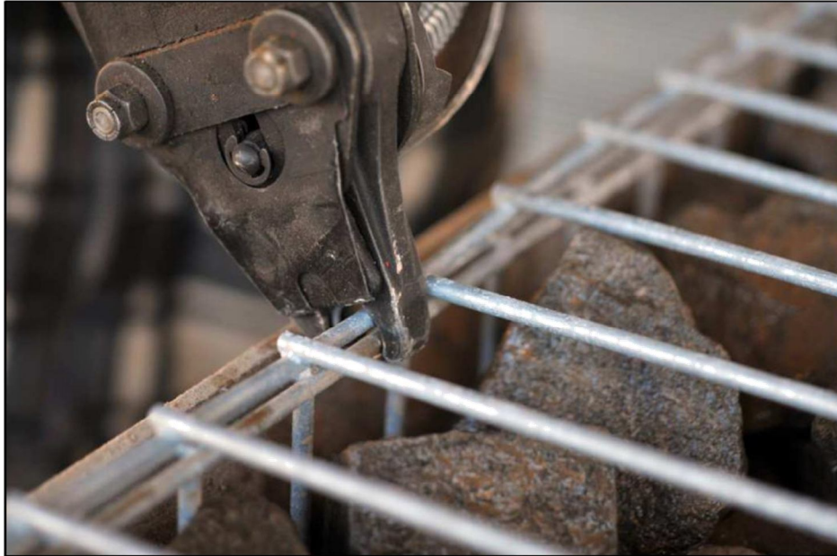
Fig.7 – Particular metal rings for the connection between covering panel and side panels –
